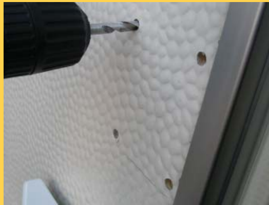
Drill 2 x 4 holes 7mm diameter.
