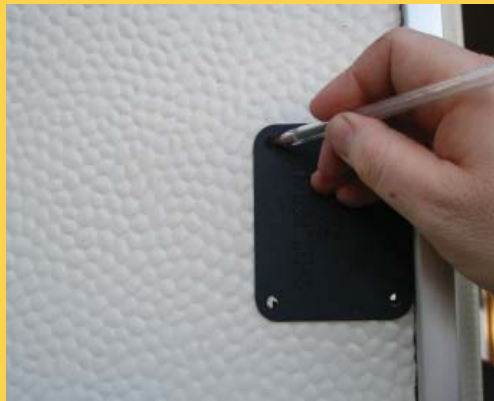
Use Gasket to mark drill position. Double check distance between top and bottom mounting points.
