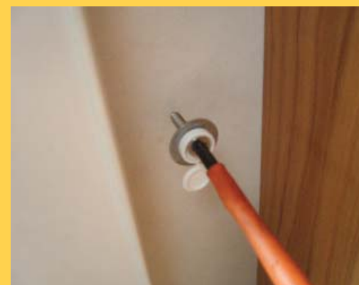
Screw base from behind in 2 places.
