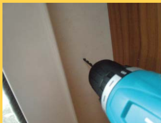
Check position of base and drill centrally.
