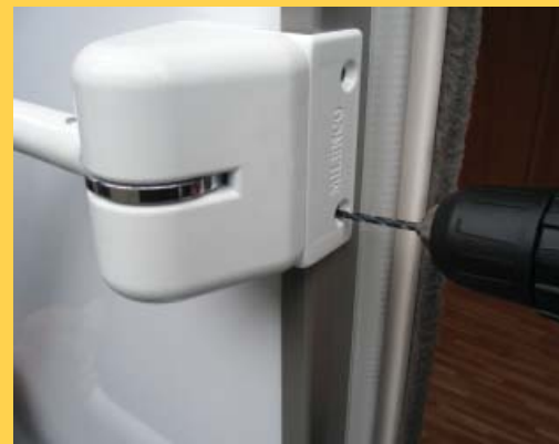
Drill 4 holes 4.5 dia.
