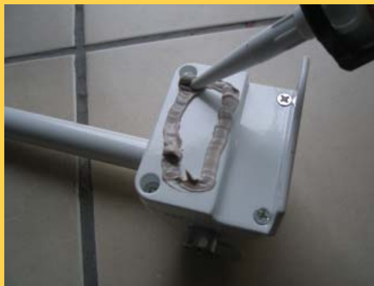
Apply sealant to base.
