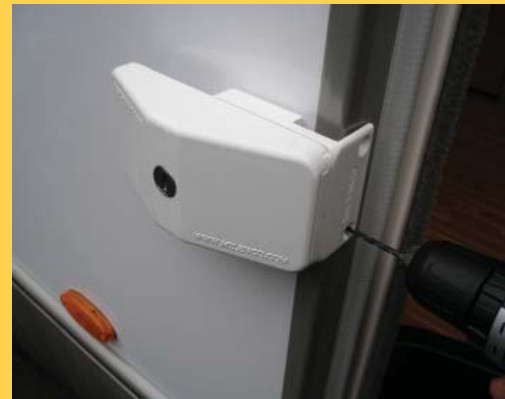
Drill 2 holes 4.5 Diameter
